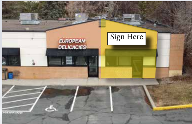
Front Facade of Suite 11040
